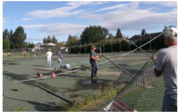
TAKING DOWN THE FENCING AND CUTTING OUT POSTS
