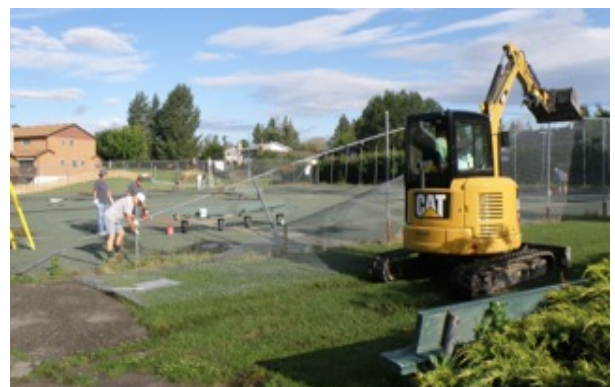
TAKING DOWN THE FENCING AND CUTTING OUT POSTS
